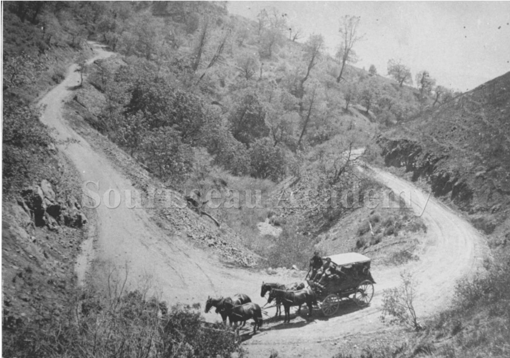
[4] Resting the Horses ... - The roadway reputedly incorporated 365 hairpin turns, depending on who was counting. Engineers and surveyors designed the right-of-way with less than a 6\frac{1}{2}\% grade so that heavily loaded, horse-drawn wagons could ascend the mountain roadway. Even today, the steep grade and narrow roadway make driving difficult.
