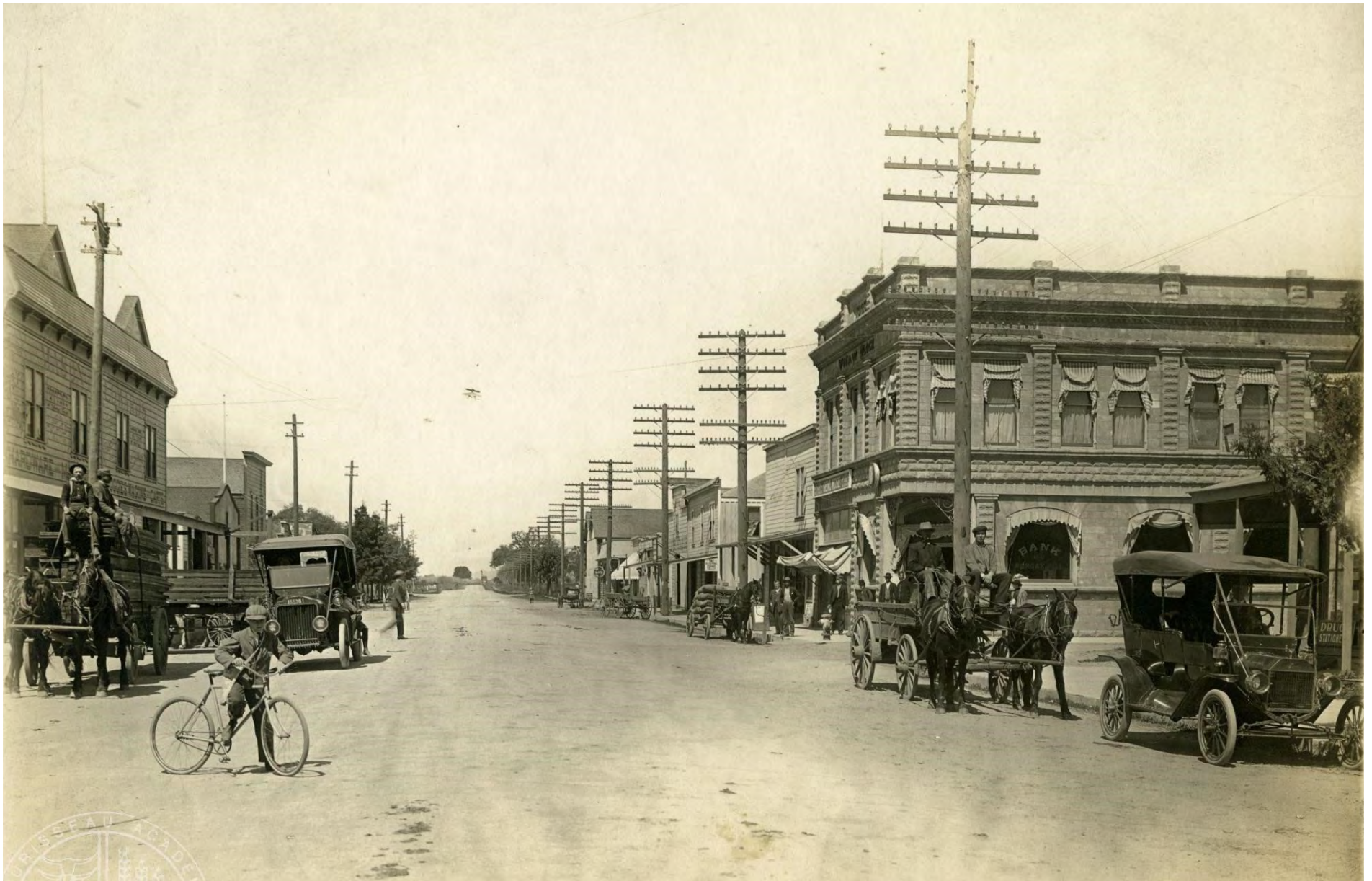
[60] Bank of Morgan Hill, 1908. Designed by San Jose architects Wolfe & McKenzie, construction of the two-story Bank of Morgan Hill was begun by the Votaw brothers in 1905. At the time of the San Francisco earthquake on April 18, 1906, the second story was unfinished and collapsed into the street, requiring the bank to be rebuilt.
